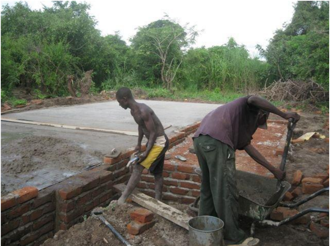
The work on the solid foundations for the new school building
