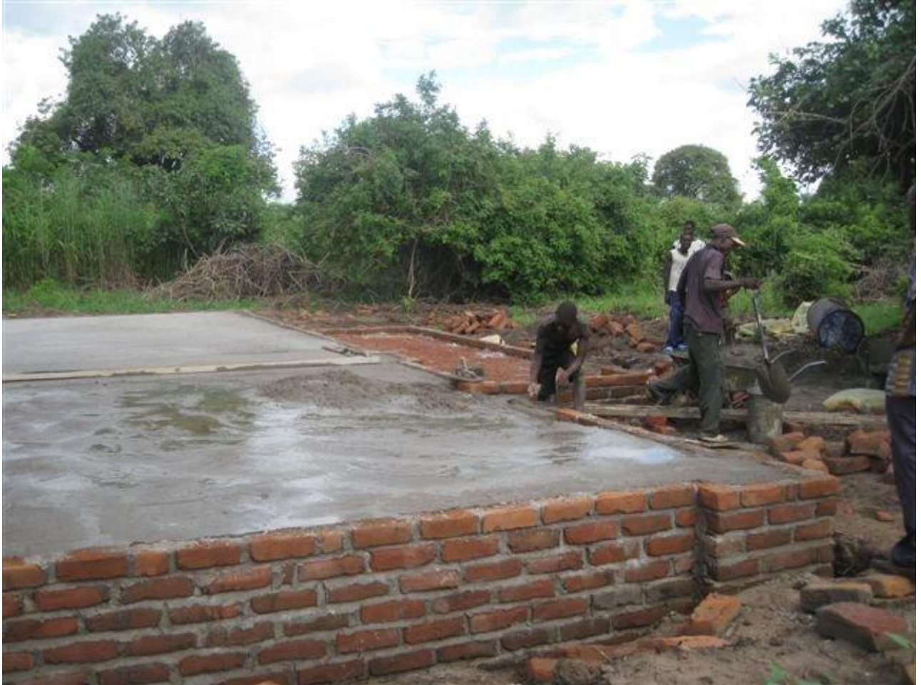
50 cm deep foundation - a good start for the new building.
