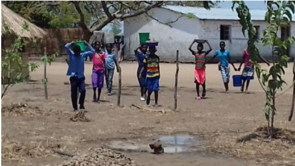
Pupil volunteers bringing stones for the building of the cement surround and runoff
