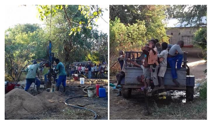
Drllling finished, casing in – installing the gravel pack filter.
