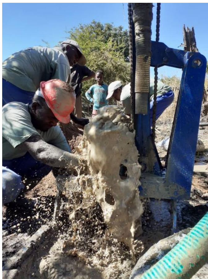
Flushing the casing in
