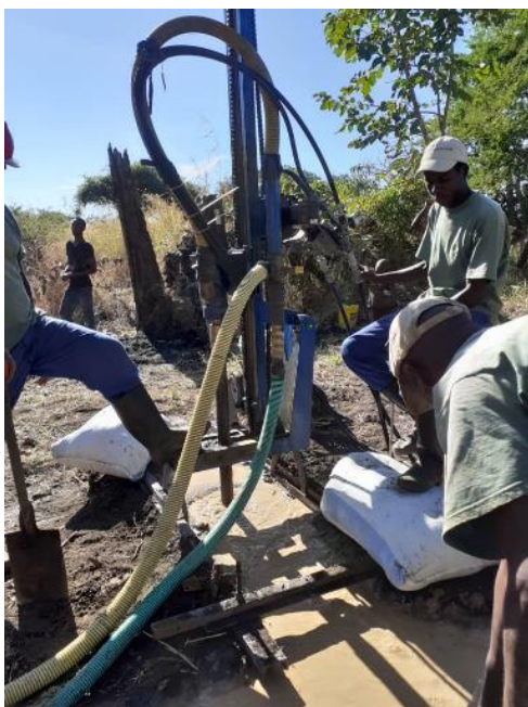
Rig and drilling team in action
