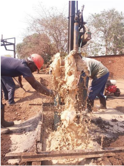
Putting in the casing at Kalumba.
