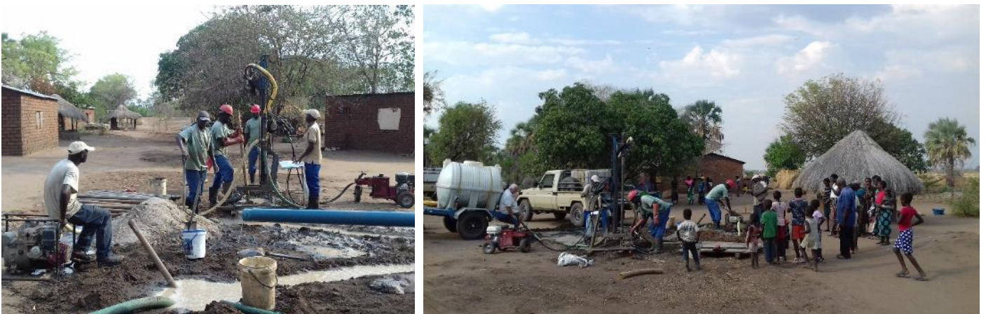
Drilling underway at Kalumba Village
