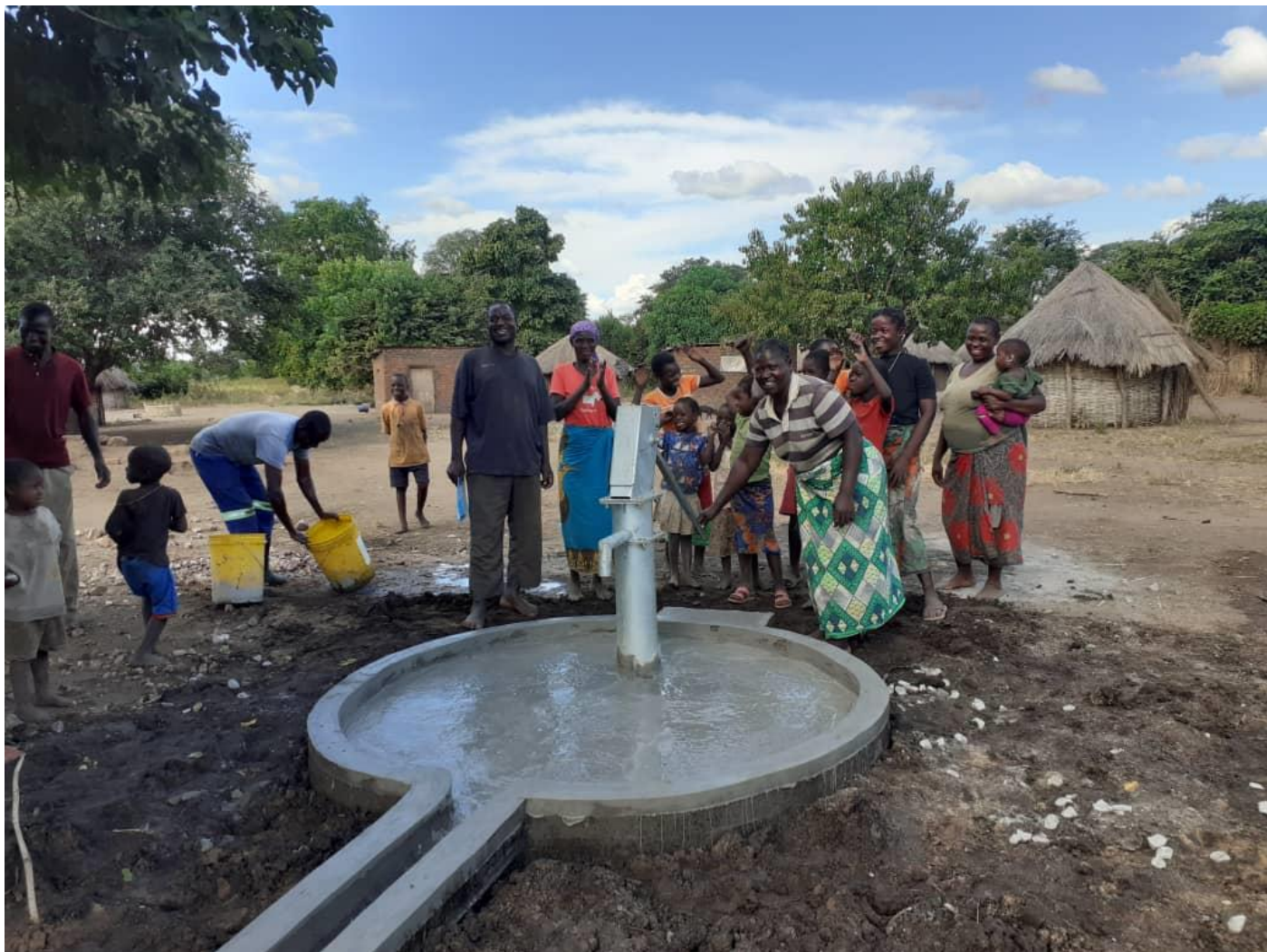
Headman Gesani delighted as the first water is pumped from the brand-new hand pump – no more dirty water for his community!
