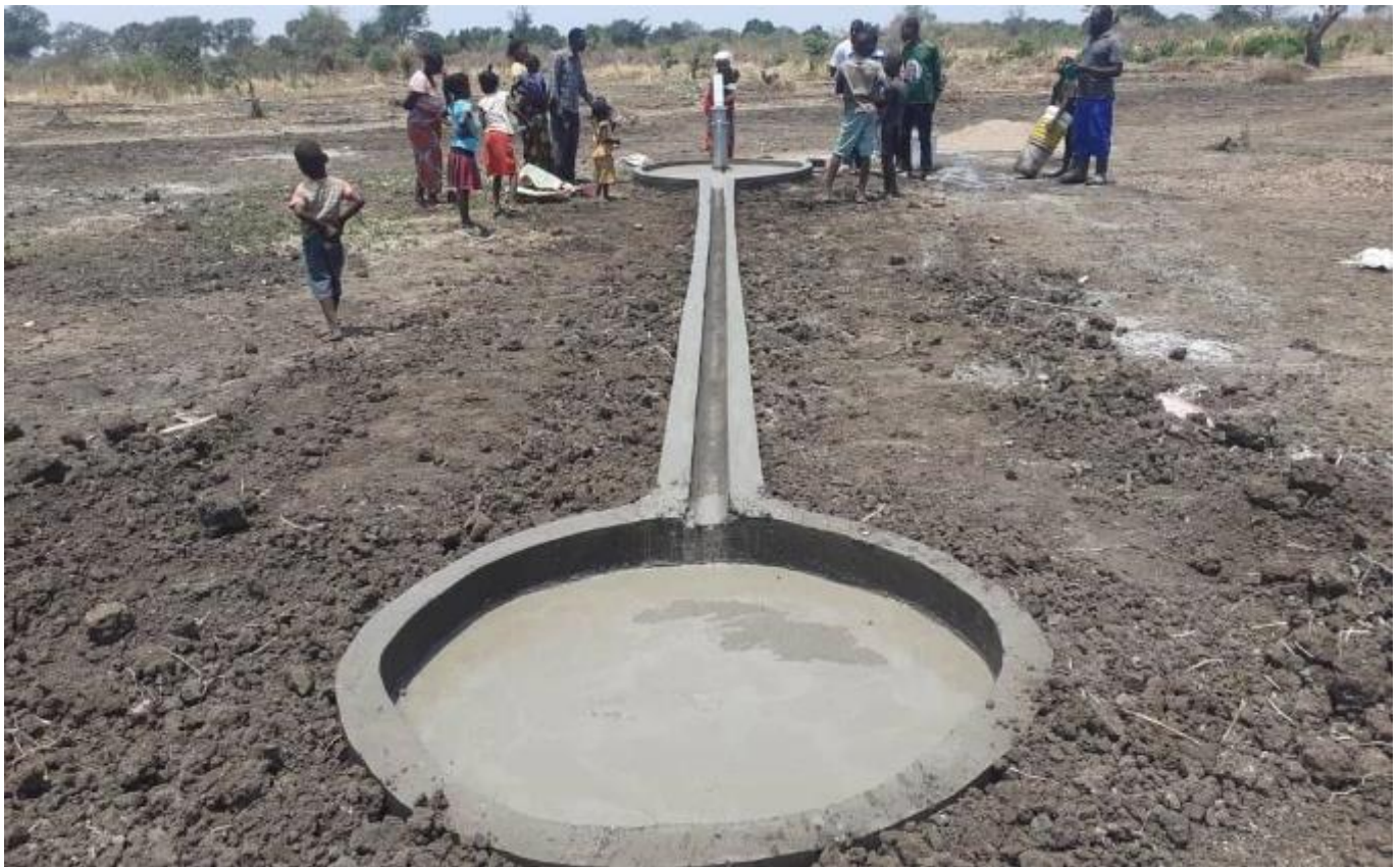
Waiting for the concrete to dry at Kambwi – this pic clearly shows the ‘garden pond’ feature.
