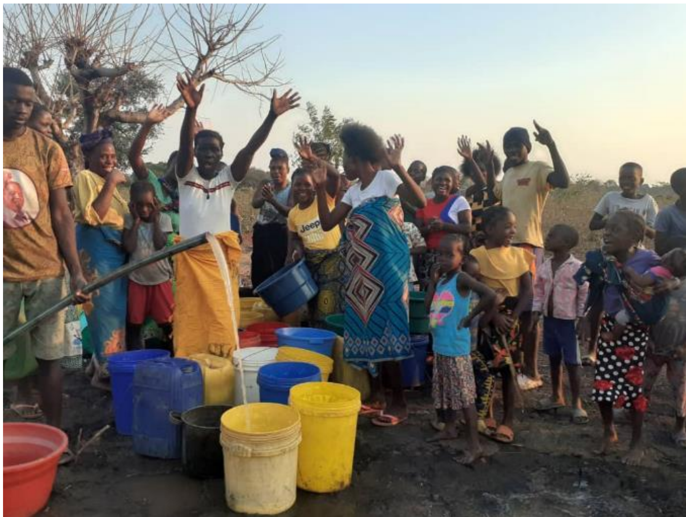
Pump testing is always a real highlight as the first water flows! Some good news after the tragic times Kambwi residents have endured.
