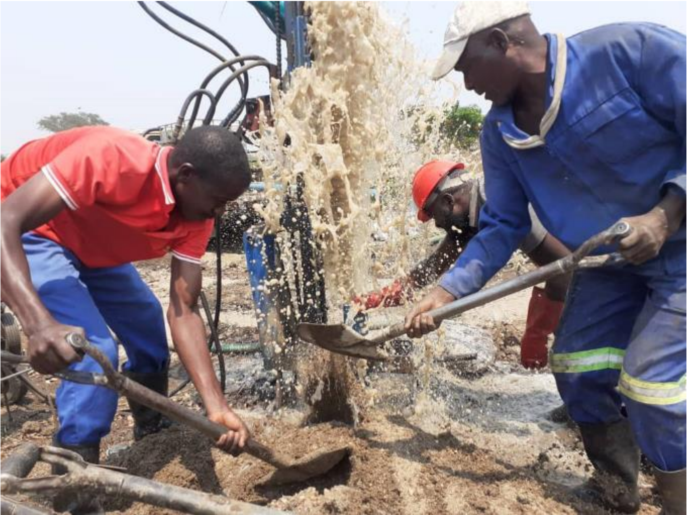
Drilling at Nguleta HQ
