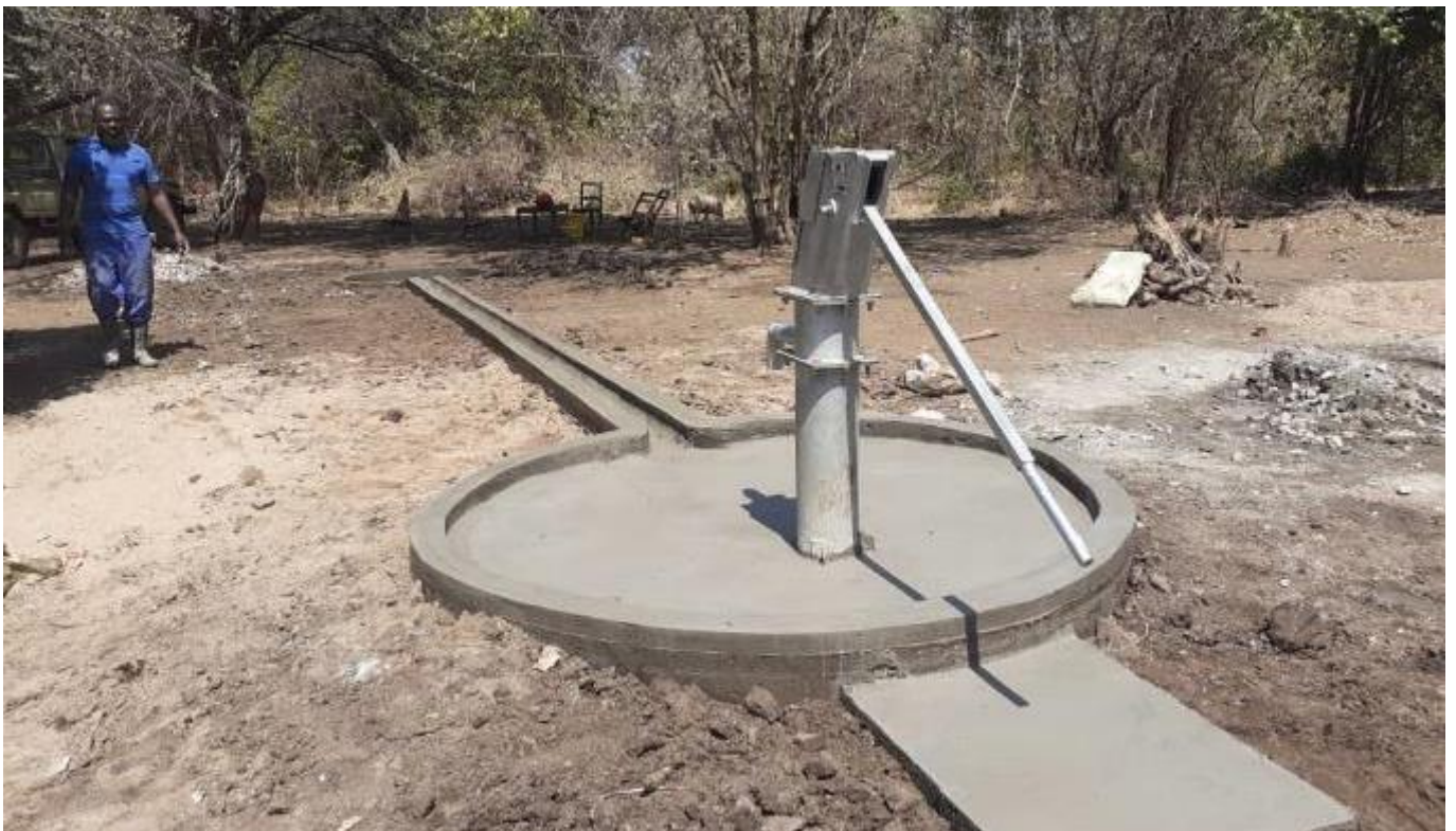
The India Mark 2 handpump installed
